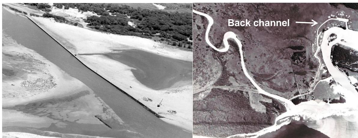
**Figure 4.16.** Armoring of the lower St Lucia estuary banks with cement-sand bags and dolosse (left, 1976) and the back channel excavated in 1970-71 (aerial photo from 1976) (Source: Illenberger & Clark 2014).
